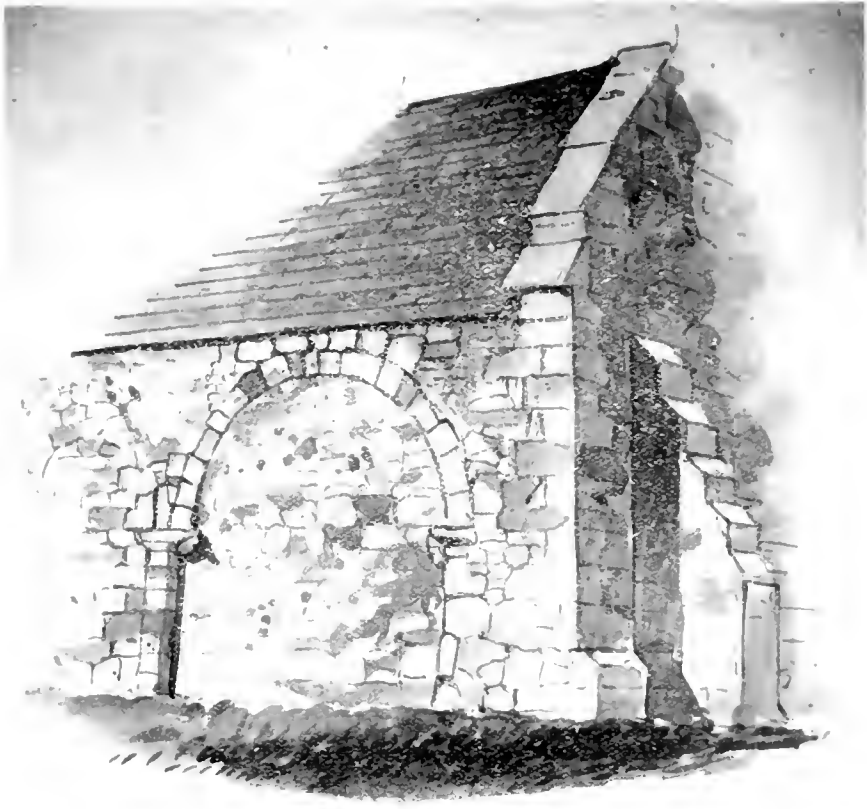
FIG. 24.—LLANDRINIO: THE PARISH CHURCH (No. 364). EXTERIOR, SHOWING NORMAN ARCH.
